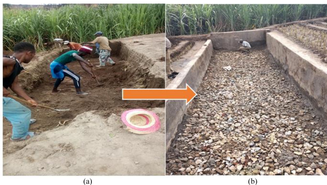
Figure 6. Construction of open space between 2 wetlands: (a) during excavation and (b) after construction.
