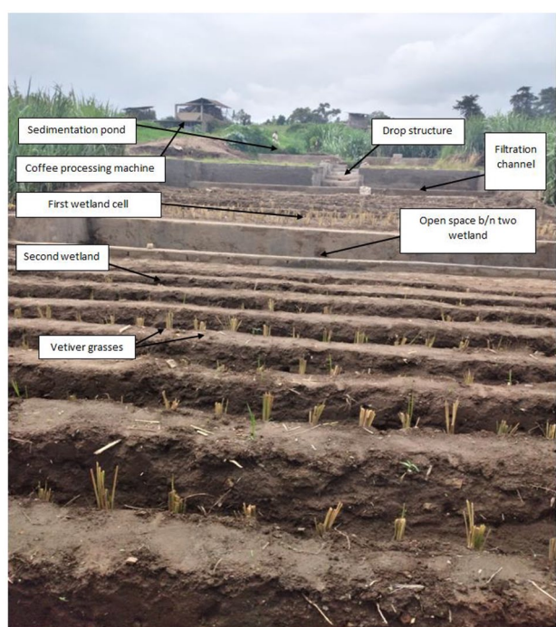
Figure 10. Whole system of wetland.
