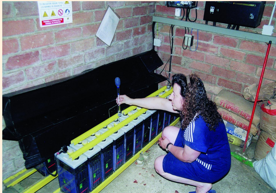
FIGURE 3 A user confidently checks the batteries of a stand-alone system in the Pyrenees. (Photo by TTA)
