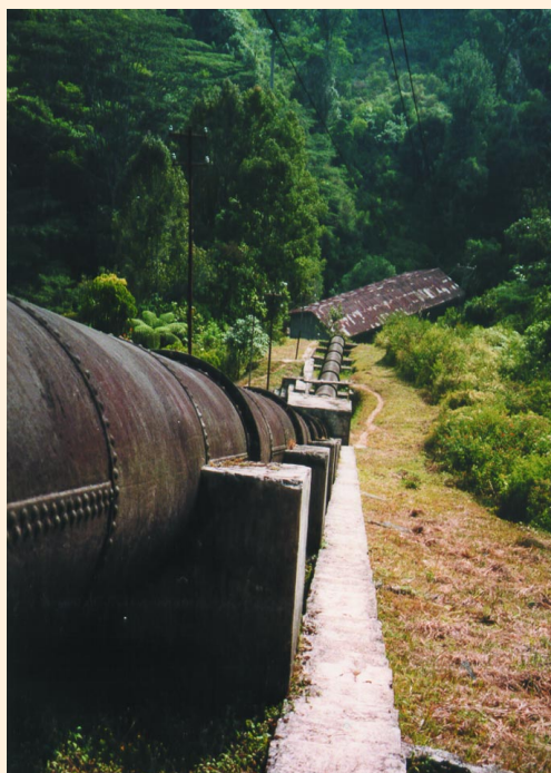
FIGURE 6 The impressive power plant at Malabar (1.5 MW). Though still running, it urgently needs renovation. Hopefully, this historic plant will benefit from the renewed interest in hydropower and remain operational for another century. (Photo by Sven Darnedde)
