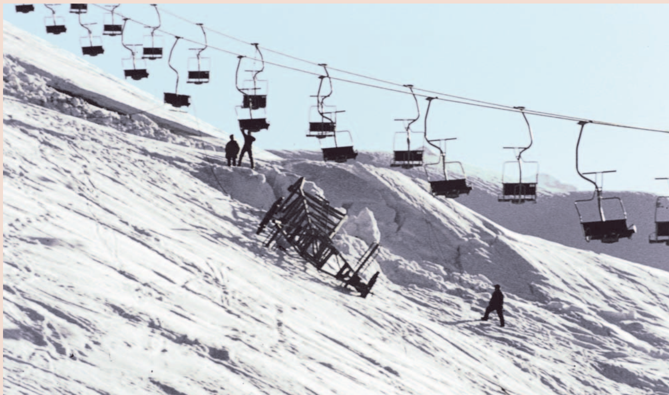
FIGURE 3 Chair lift pylon damaged by snow pressure on 14 March 1999, in Hasliberg (Canton of Berne, Switzerland). (Photo courtesy of SLF)
