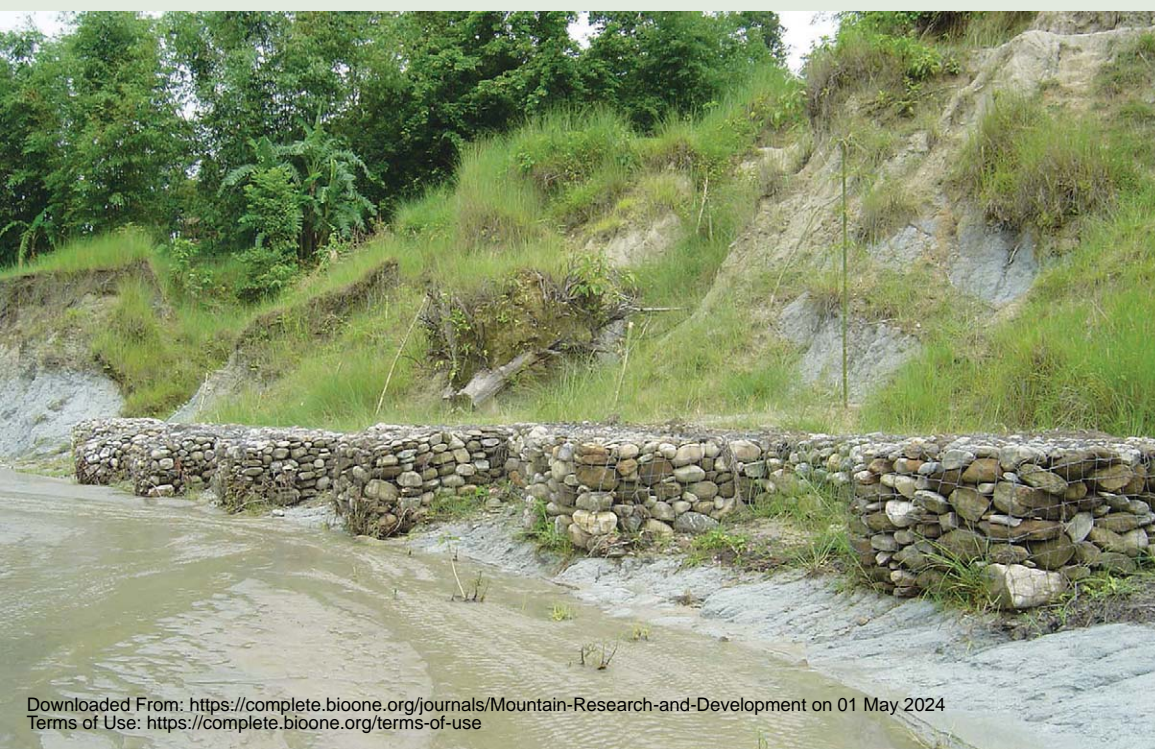
FIGURE 1 Community-managed spurs to protect the land from seasonal floods. (Photo by Ram Chandra Khanal)
