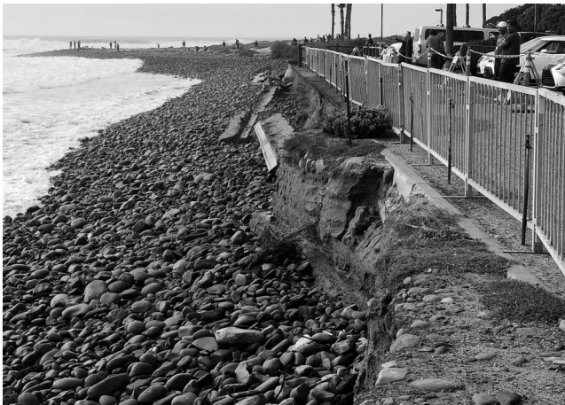
Figure 11. Erosion of the bike path and bluff along the Promenade in Ventura California during the large wave event of January 9th, 2019.
