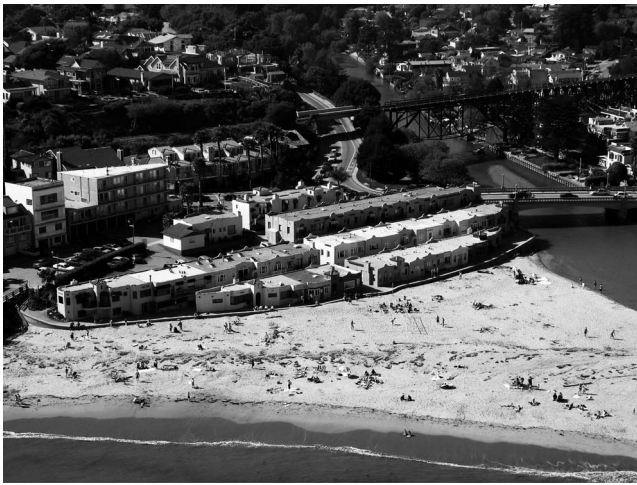
Figure 6. The Venetian Court condominiums, built essentially on the beach in Capitola in 1923, are repeatedly flooded by the combination of storm waves and high tides.
