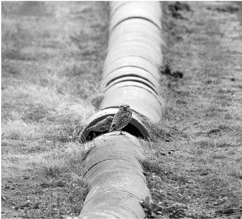
Figure 1. Burrowing Owl perched outside nest burrow entrance into concrete half-round cable cover, National Radio Transmission Facility, Dixon, California.
