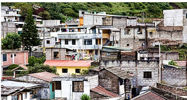
Figure 6. Local architecture characterized by poor ventilation in Ecuador (Belsky, 2023).
