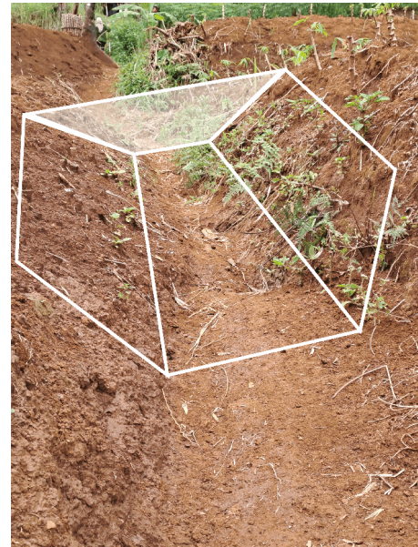
Figure 5. Shape of rill erosion.
