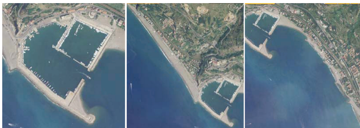
Figure 4. Aerial view of the actual situation of Cetraro Port, of the northwest side and of the southeast side.
