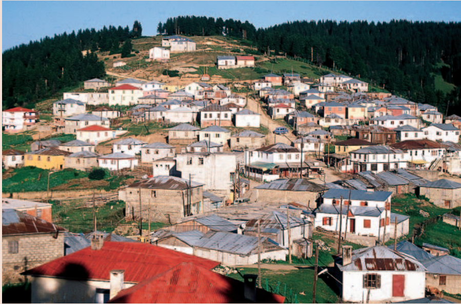
FIGURE 2 Although Turkish law only allows the building of temporary dwellings in the highlands, an increasing number of permanent homes have been constructed, using non-traditional material and architecture. The village of Kumbet in the Black Sea region. (Photo by M. Resat Sümerkan)
