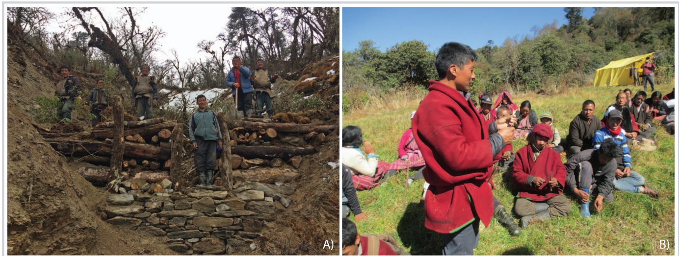
FIGURE 3 Project activities included, among others, (A) check dam construction with herders and (B) social learning on pasture improvement. (Photos by Norbu Yangdon and Joanne Millar)
