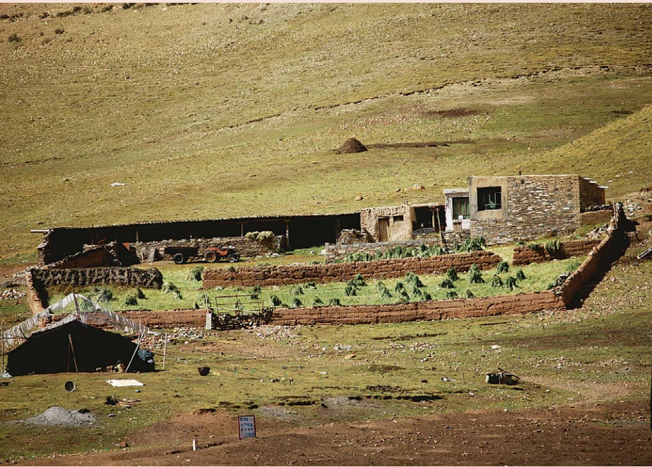
28 FIGURE 2 The “Four-Way Scheme” policy: a winter house, livestock shelter, fence (wall), and winter fodder are shown here, along with a traditional tent in the foreground. (Photo by author)
