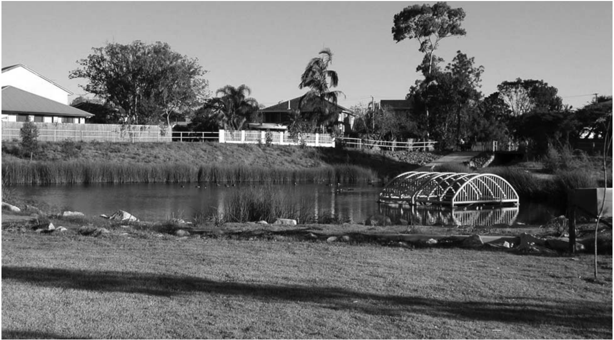
Sedimentation basin as an inlet zone for a constructed wetland.
