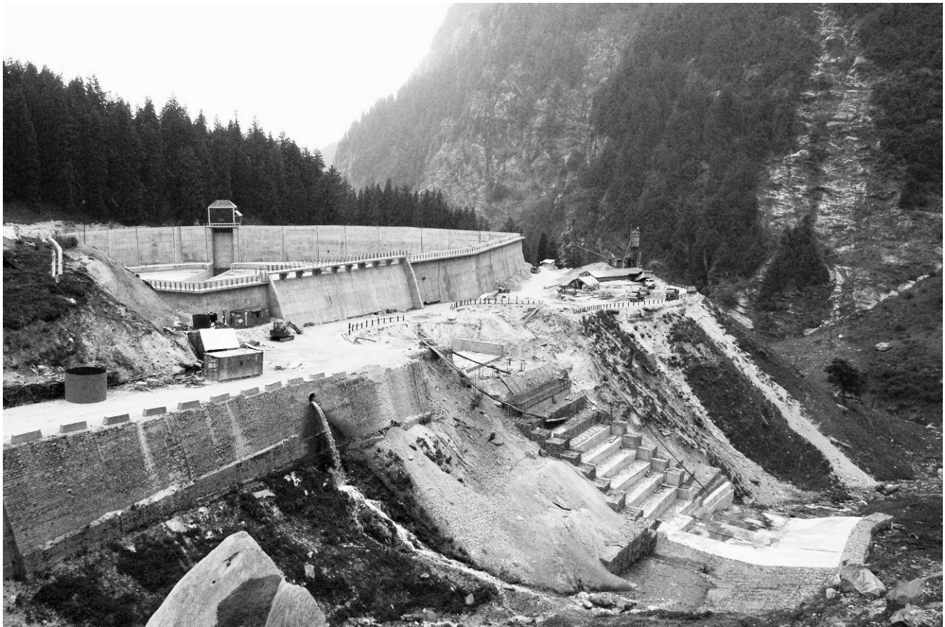
FIGURE 2 Allain Duhangan intermediate reservoir under construction. (Photo by A. Erlewein, 13 June 2009)
