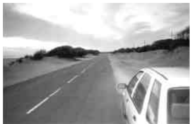
Figure 2. Existing road alongside La Bota beach (Huelva, Spain), Gómez-Pina 1997.
