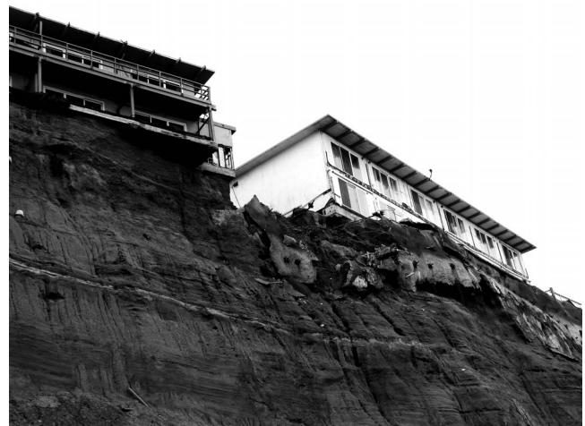
Figure 13. These apartment buildings in Pacifica were built on a high eroding bluff in the early 1970s, and despite efforts to protect them, they were declared unsafe to occupy and then demolished in 2016.
