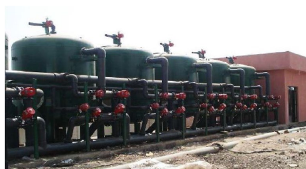
Figure 9. Rapid sand filters following the Oxidizer at Bani Murr WTP to filter out the oxidized iron and manganese.
