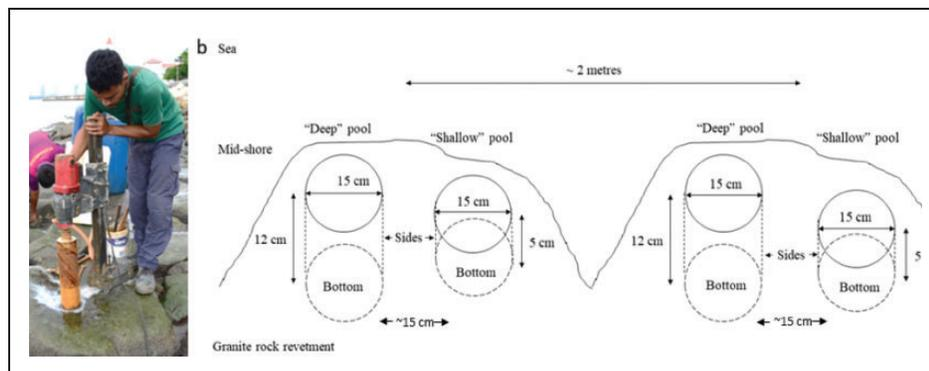
**Figure 3.** (A) Drill-coring 15 cm diameter artificial rock pools into horizontal granite surfaces of rock revetments at Straits Quay Marina, using a diamond-tipped drill corer. (B) Cross section view, dimensions, and arrangement of drill-cored artificial rock pools on granite rock revetments at study sites. Emergent surfaces were dispersed in between the rock pools.
