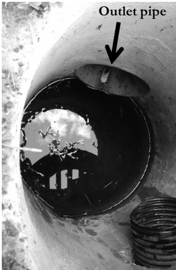
Figure 3. Evidence of catch basin larvicide flushing. A Natular™ XRT tablet is observed sitting within a catch basin's outlet pipe after initially being placed within the basin's sump water below.
