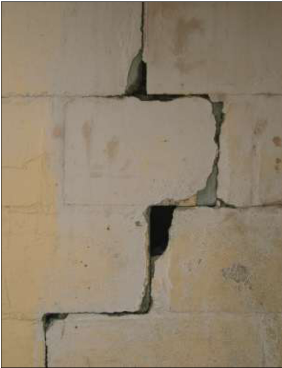
Figure 4. An example of structural damage: a seriously cracked wall of main house in Tafelsig.
