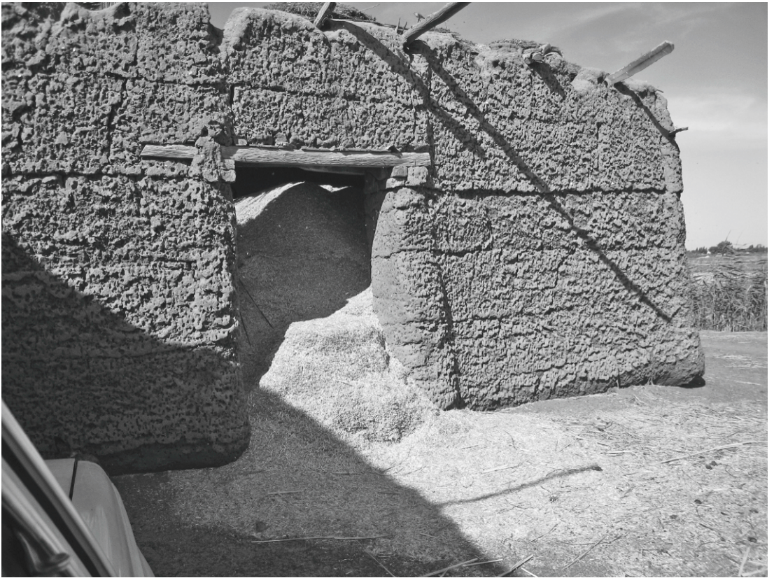
Fig. 2. The grain storage building at El-Huseiniya, site 4. Note erosion of adobe wall caused by nesting bees and hood of white pickup truck, lower left; see text for explanation.
