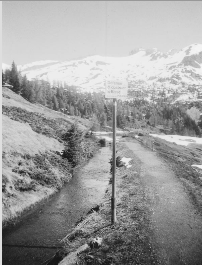
FIGURE 1 An open bisse or irrigation channel that conveys water for summer pastureland in the highly developed agricultural and tourist area of Montana-Aminona, Canton of Valais. Translated into English, the sign reads "Obstructing the bisse is prohibited." (Photo by author)
