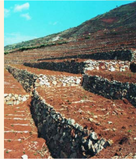
FIGURE 2 Bench terraces have been promoted extensively as a soil conservation measure, but they require a high level of investment for construction and maintenance. (Photo by Tang Bo)
