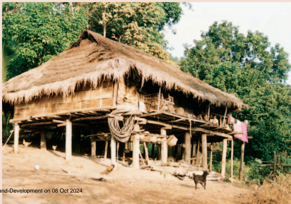
FIGURE 1 A traditional Karen house, Pae Por Highland Development Project. (Photo by author)
