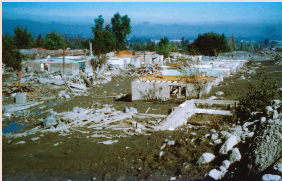
FIGURE 4 Devastation resulting from the flash flood of 3 May 1993 in Macul watershed. (Photo by Francisco Ferrando)
