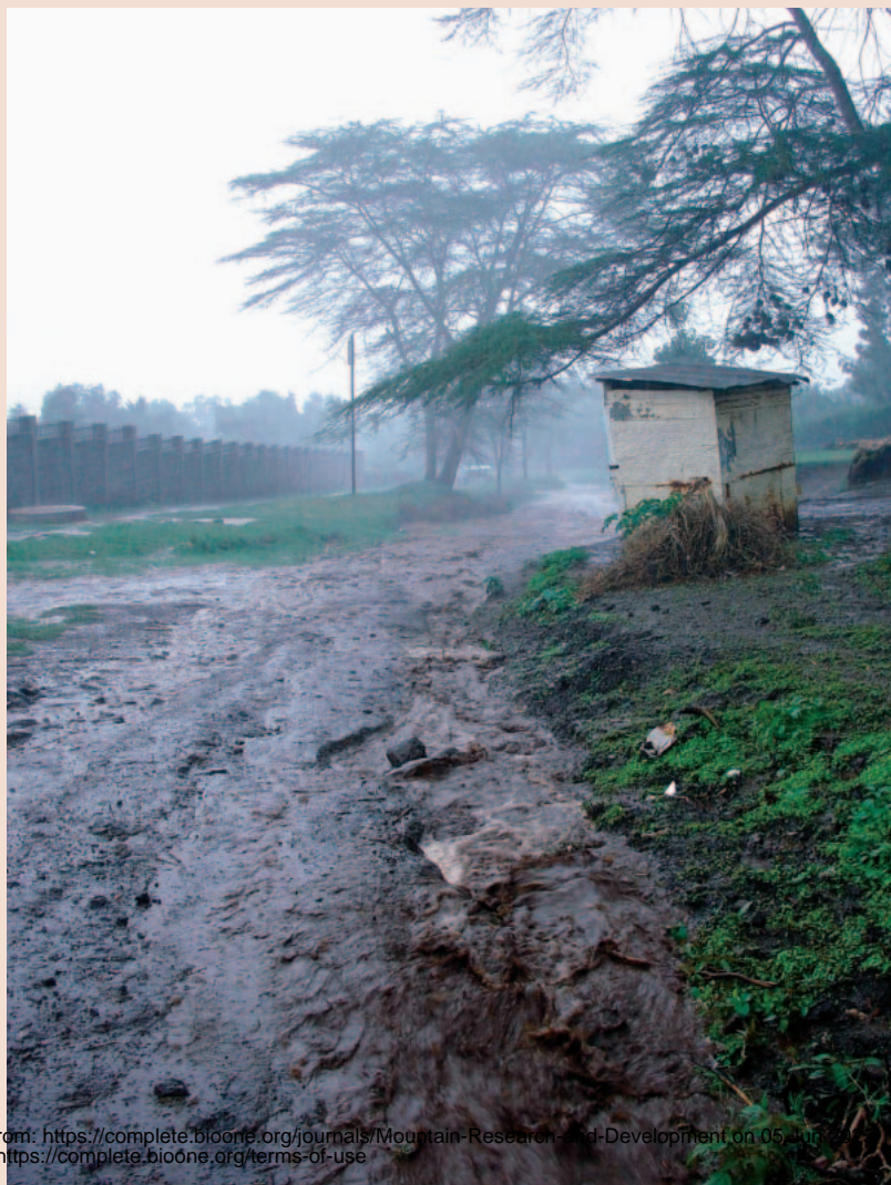
FIGURE 3 After every heavy rainfall (a daily occurrence in the rainy season), this road leading to the crater is transformed into a river. The sediment-loaded water reaches high speeds and carves deep gullies into the road, rendering it impassable at times. The fragile volcanic soils are washed away as a result of deforestation, inappropriate land use practices and overgrazing. (Photo by Albrecht Ehrensperger)
