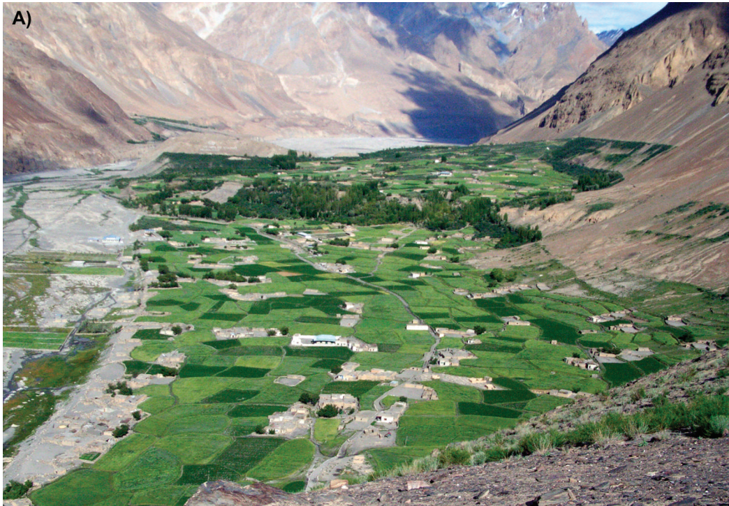
FIGURE 3 (A) Shimshal center in July 2007 with the new road bisecting the settlement. (B) A difficult section of the route to Shimshal, showing the old footpath and the partially completed road. The photo was taken in July 2000, when this section of the road was being constructed. (Photos by David Butz)
