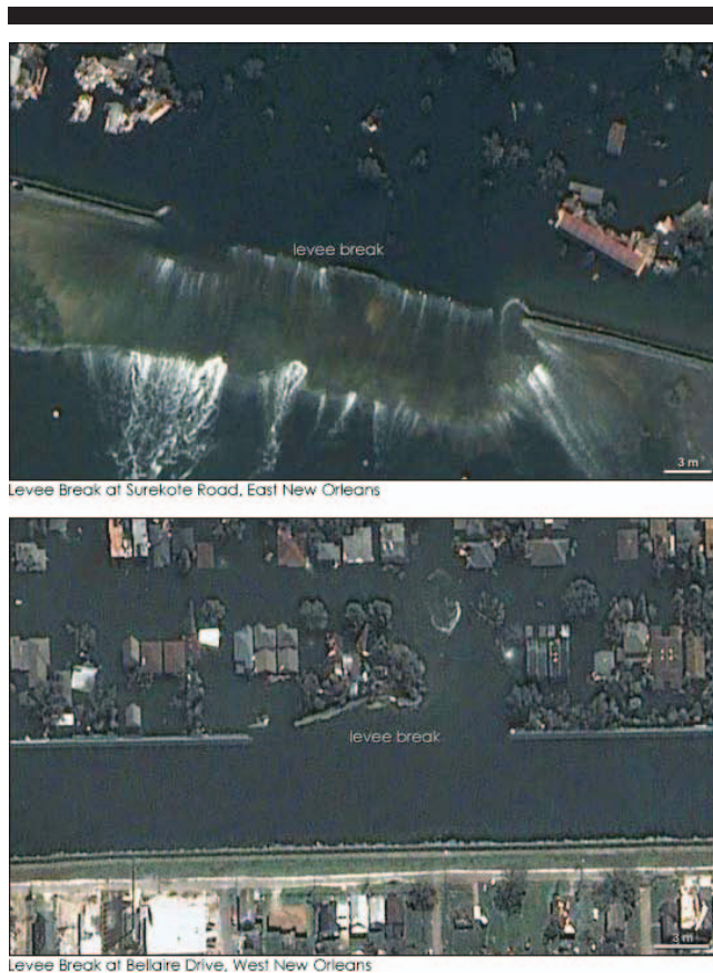
Figure 6. QuickBird satellite images of New Orleans levee breaks (Digital Globe, 2005).
