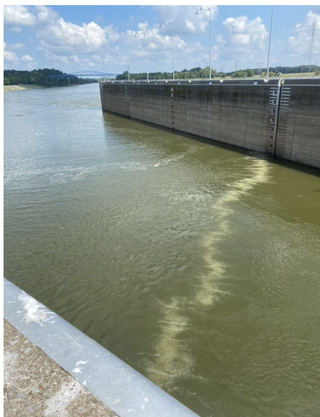
Fig. 3. An experimental BioAcoustic fish fence (BAFF) in operation at the downstream approach channel of Barkley lock on the River Cumberland near Grand Rivers, Kentucky. Photograph shows the air-bubble curtain when the system is turned on. The BAFF is planned to be operated for up to three years for a research study to evaluate its effectiveness to reduce upstream passage of invasive carps.
