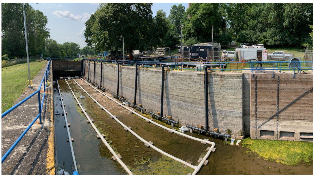
Fig. 4. Installation of an experimental carbon dioxide (CO 2 ) deterrent system at lock #2 on the River Fox near Kaukauna, Wisconsin. Photograph shows gas distribution piping on bottom and side of lock chamber. This system was temporarily installed for research purposes in 2019 to evaluate gas system engineering and performance within navigation lock chambers.
