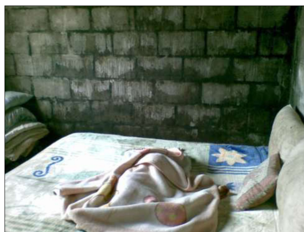
Figure 3. Dampness penetrating bedroom wall with infant sleeping on bed in a low-cost house in Greenfields.
