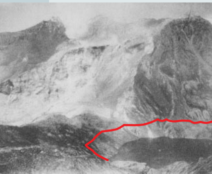
FIGURE 2 View toward the southeast from the top of the Usoi dam, Lake Sarez, in about 1940. The line shows the approximate level of the water in 1992. (Photo courtesy of S. F. Cunha)
