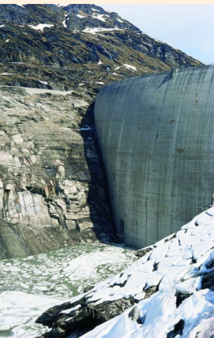
FIGURE 6 Reservoir management and sediment flushing: The Zervreila dam (Switzerland) was completely emptied for maintenance work in the 1980s. Careful procedures must be followed in operations such as this as well as in periodic flushing to remove sediment in order to minimize downstream ecological impacts. (Photo by B. Wehrli)
