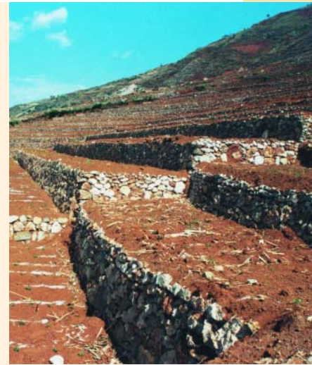
FIGURE 2 Bench terraces have been promoted extensively as a soil conservation measure, but they require a high level of investment for construction and maintenance. (Photo by Tang Bo)
