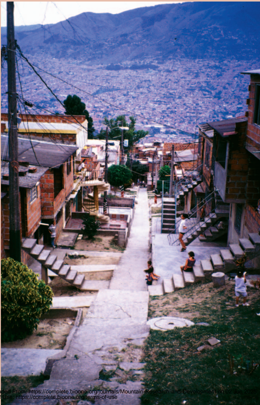
FIGURE 1 Public social housing built in the 1970s. During the following decades, people enlarged their houses by building a second floor. The houses in these planned districts are accessible only via steps and paths meant to stabilize the soil. But contrary to planners' advice, the paths have been built perpendicular to the slopes, in alignment with the grid structure of the city. (Photo by Angela Stienen)
