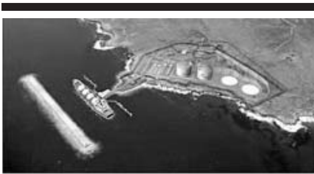
Figure 3. An aerial photograph of the newly constructed LPG terminal at Costa Azul, Baja, Mexico, which was constructed on top of world class surfing resource. (Source: Save the Wave Coalition, 2006)
