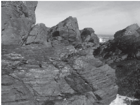
Large rocks with cracks
