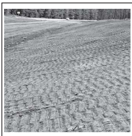
Figure 5. Trackwalking is often used to increase slope stability, but will compact both surface and subsurface soils.
